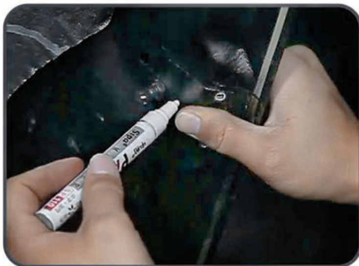
2. Confirm the drilling location on the hood
